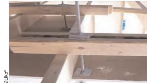
Figure K-11: Threaded Rod Mount
