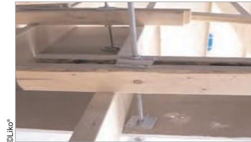
Figure K-11: Threaded Rod Mount
