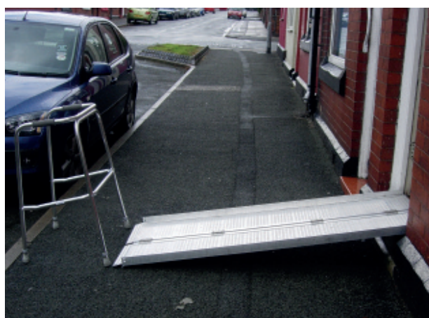
Figure 4 Long ramp to reduce the incline
